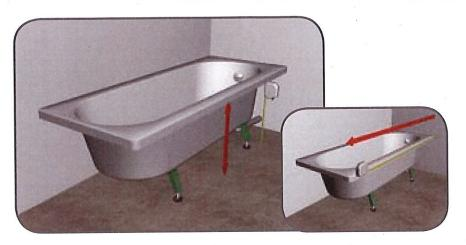
**Step 10**Measure the overall length required from wall to end of bath. Measure the overall height from the floor to the underside of the bath.
