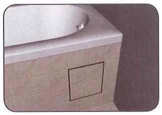
**Step 1**Establish the quantity of tiles required to allow adequate access and remove the grout around the area.
