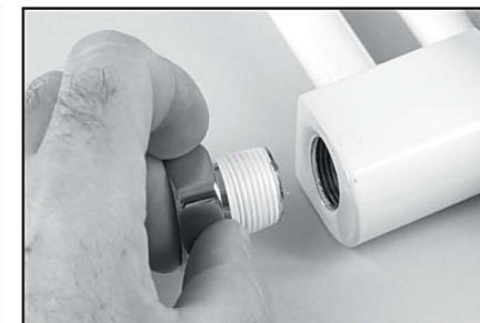
2. Screw the threaded end into the radiator or towel rail
