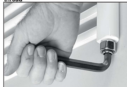
3. Tighten using an appropriate tool
