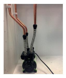
**11** When everything is watertight, open any outlets so that a natural flow under gravity can fill the system, it can be plugged in, or the plug removed and wired into a fused spur so that the pump can be fully tested.
