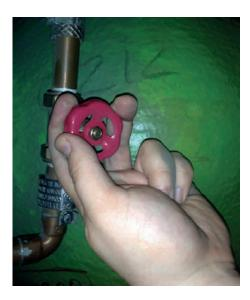
**5** The existing push - fit hoses can now be removed by pushing the gripper ring towards the hose and sliding the body away from the pipe - depending on the installation the outlet hoses may be suitable for the new pump without changing them.
