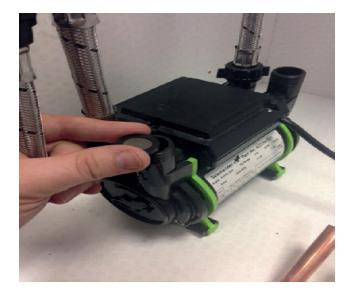
8 Once the pump and hoses are in place, it will be possible to mark or measure how much of the inlet pipework will need to be trimmed back using a pipeslice or cutter.
