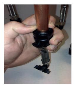
The new pump can now be unpacked, the noise reducing rubber feet fitted and the pump offered up to the installation - if the installation will allow, the outlet flat washer can be fitted and the pump connected to the outlet pipework. If the installation will not allow this, the new, longer hoses may be used following the next steps...
