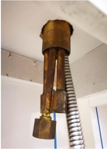
Step 3: Put the tap through the sink
