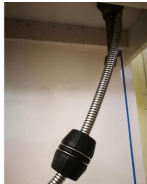
Step 7: Put the Weight onto the hose
