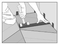
**8.** Cut the final row of planks to fit along the wall. Use a pull bar to lock the long edges together. Do not use the pull bar on the short edges.
