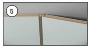
Starting at approximately 45°, angle the tongue of the next panel into the groove of the fixed panel. Ensure the tongue is fully inserted into the groove before snapping it back to the wall, otherwise it may damage the joint.
