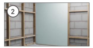
Bond the first panel to the wall or frame, with the grooved edge first. If screw fixing panels to the wall/ frame, pilot bore the recess in the groove where screws are to be located. Failure to pilot bore may result in the panel's joint splitting). Pack between back of panel and wall as necessary to avoid distortion to the Hydrolock joint when screw fixing and to ensure that it is true and plumb.
