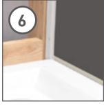
Apply high grab adhesive to the reverse of the Multipanel® angle into the first profile and push firmly against the wall.
