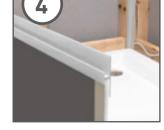
Apply silicone sealant to the channel of the second profile and attach it to the long edge of first panel.
