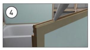
Apply masking tape to the two meeting edges of the decorative face to protect the laminate face. Apply a narrow bead (2-3mm) of silicone sealant to the front shoulder of the tongue.
