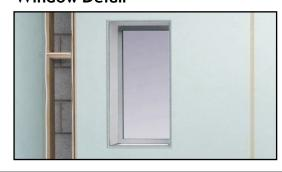
At windowsills, a Type E quadrant end cap should be used between panels, and mitred in the corners.
