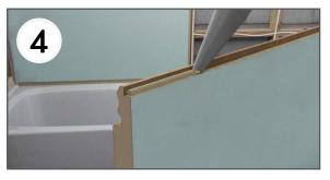
Apply a narrow bead (2-3mm) of silicone sealant to the front shoulder of the tongue.
