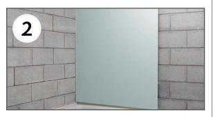
Bond the first panel to the wall or frame, with the grooved edge first. If screw fixing panels to the wall/frame, pilot bore the recess in the groove where screws are to be located. (Failure to pilot bore may result in the panel's joint splitting). Pack between back of panel and wall as necessary to avoid distortion to the Hydrolock® joint when screw fixing and to ensure that it is true and plumb.
