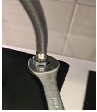
The inner seal may come lose from inside the connector. Make sure to place this seal back inside the connector.
