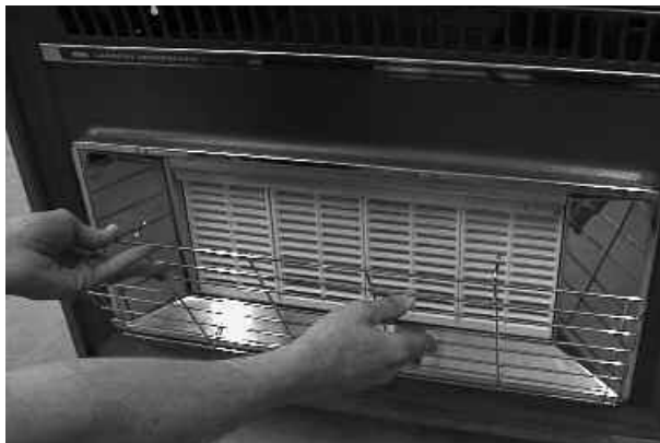
Fig. 2 Remove the Dress Guard.
