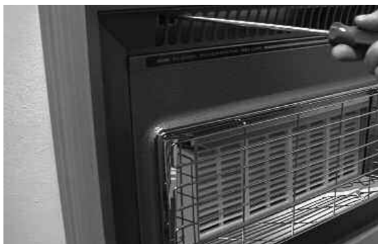
Fig. 10 Removing the Upper Outer Case Fixing Screws
