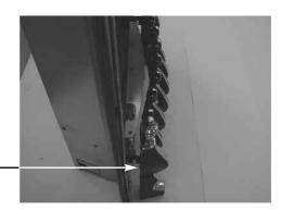
Correct position of fender, located onto firebox
