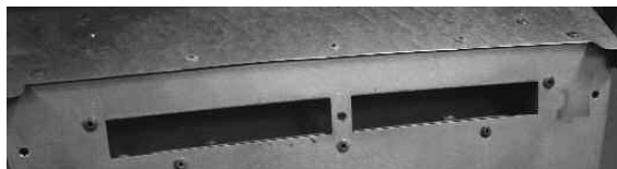
Fig 4 - Flue Restrictor Baffle Not Fitted
