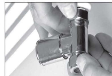
4. Attach valve and turn finger tight in to the correct position
