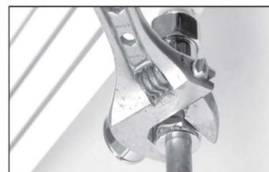
7. Tighten the the nut that holds the pipe in position
