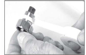
Wrap PTFE tape clockwise around the tail thread
