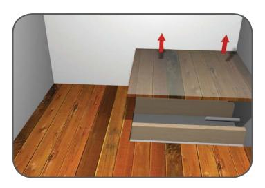
Remove flooring as necessary to carry out works to the wastepipe. Please note that if there is a joist in the way of the Shower Tray you will need to consult a professional joiner or structural engineer for advice.
