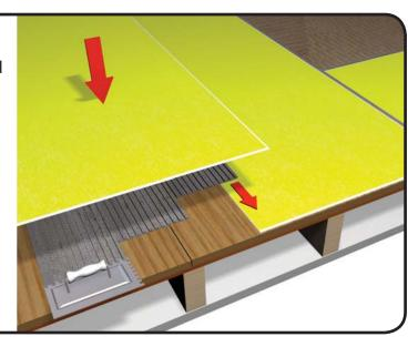
Lay the next strip overlapping the last by 50mm and repeat Steps 19 & 20 ensuring that the adhesive and matting overlaps the walls, tray and each strip by 50mm to create a waterproof seal until the floor area around the tray is tanked out.
