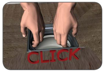
5. Put your fingers through the drain hole in the Shower Tray. Push down on the Shower Tray and pull the Shower Drain upwards until it clicks into place into the drain hole in the Shower Tray.
