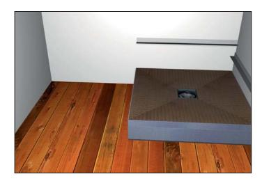
**Step 7**You will need to tape all joints where the tray meets an adjoining wall/s. Cut lengths from the roll of Waterproofing Tape and set aside for the moment.
