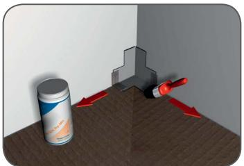
10. Place the Waterproofing Internal Corners into the internal corners of the shower area and push firmly into the Pro-SEAL tape sealer. Apply a further thin layer of Pro-SEAL tape sealer over the edges of the waterproofing internal corners.
