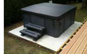
A 10-15 cm concrete base is ideal preparation for a hot tub.
