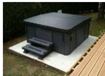
A 10-15 cm concrete base is ideal preparation for a hot tub.
