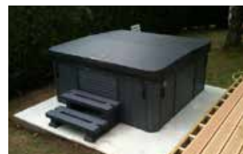
A 10-15 cm concrete base preparation for a an acrylic Plug & Play hot tub.
