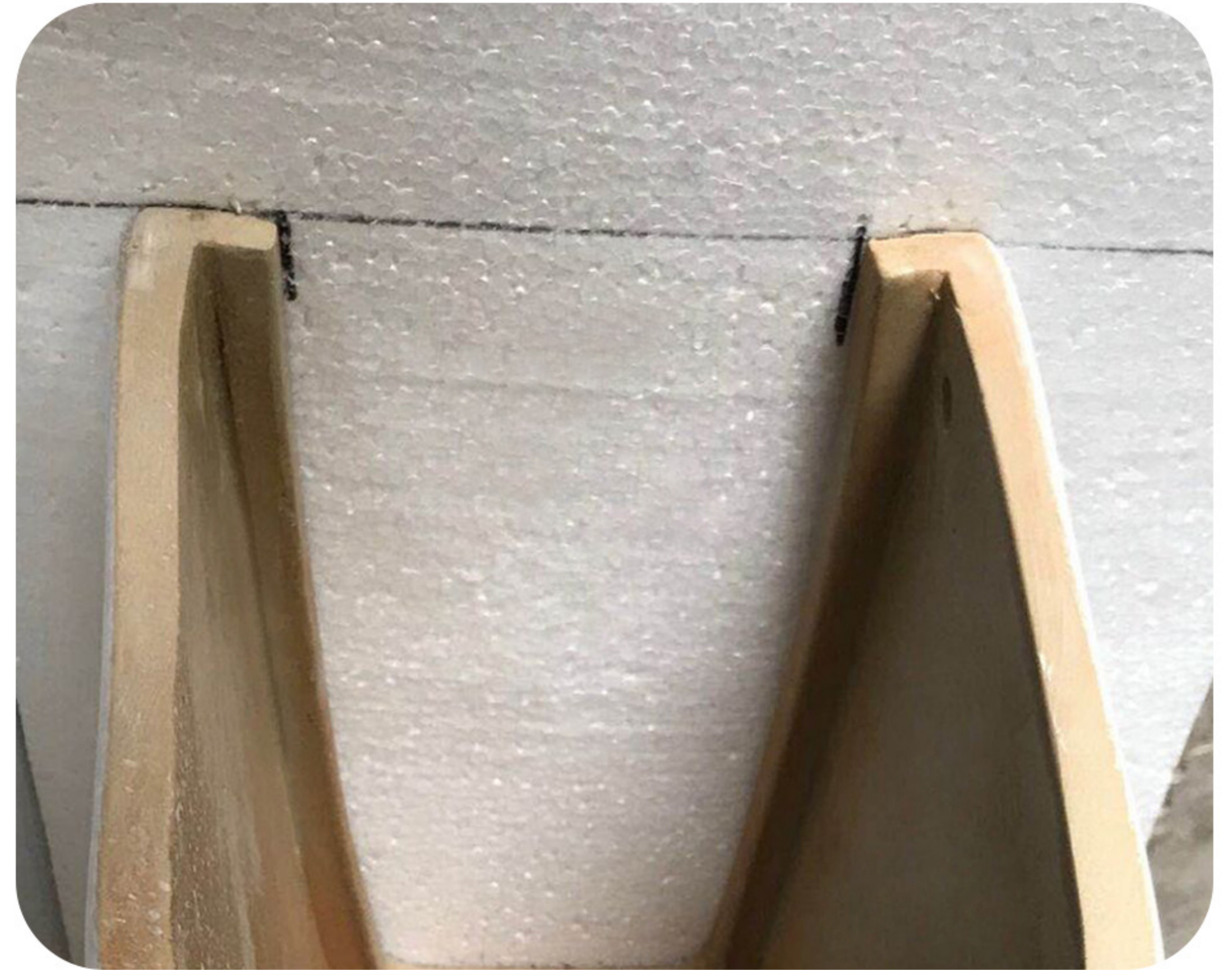
2) Put the semi pedestal on wall and mark the installation sites
