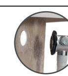
suring the rubber washer is correctly aligned, pass the overflow filler outlet through the bath and secure to the body assembly.
