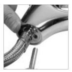
Feed the flexible hoses through the hole in the mounting surface and offer the mixer tap into position, ensuring the base O'ring remains in position. An ø30 – 35mm hole is required.
