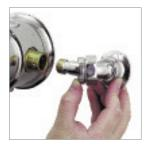
Carefully locate the elbows into the valve inlet connections and push fully home.
