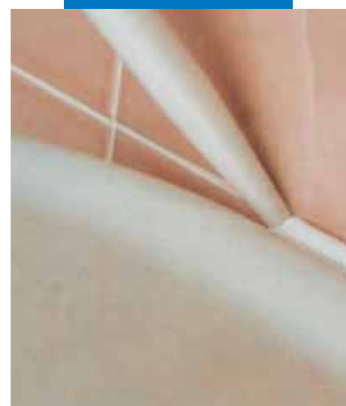
Sealing sanitary ware
