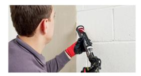
Apply a bead of ProBacker adhesive to the edge of each board to help seal and reinforce the joints. As you apply more boards, stagger the joints where possible. Keep the boards level and flat throughout.
