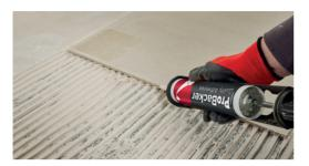
Apply a bead of ProBacker adhesive to the edge of each board to help seal and reinforce the joints.
