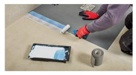
Use a tanking kit to bond all the joints and ensure these are fully waterproof. Apply the polymer adhesive with a roller between the joints and allow to dry tacky - usually after a couple of minutes.
