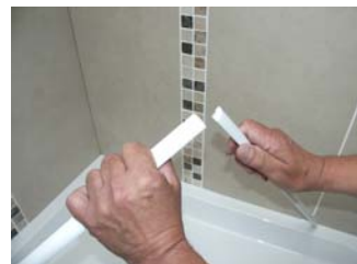
Score and snap profile - Clean with alcohol wipes and dry fit to tray to ensure they fit OK - Remove Strips and silicone tray with the large nozzle
