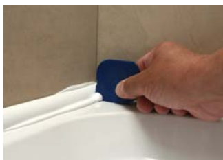
Fit profile one side at a time - push in at 45 degrees to get sealant up tiles and across tray base - Remove excess sealant with Fugi Tool or finger
