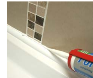
Repeat above steps - Change to fine nozzle and run fine bead along top and bottom of profile - remove excess with Fugi - Leave to Set (4 hours)
