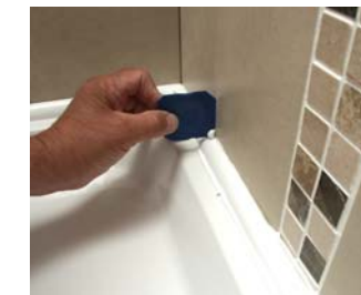
Repeat above steps - Change to fine nozzle and run fine bead along top and bottom of profile - remove excess with Fugi - Leave to Set (4 hours)
