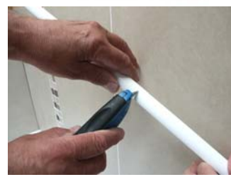
Measure tray internals and transfer measurements to profile - Mark and cut non profiled ends only
