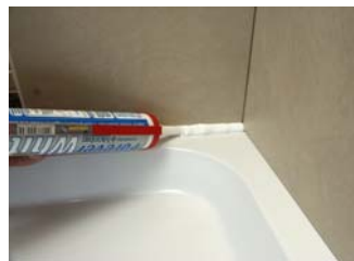
Score and snap profile - Clean with alcohol wipes and dry fit to tray to ensure they fit OK - Remove Strips and silicone tray with the large nozzle
