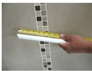
Measure tray internals and transfer measurements to profile - Mark and cut non profiled ends only
