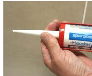
Repeat above steps - Change to fine nozzle and run fine bead along top and bottom of profile - remove excess with Fugi - Leave to Set (4 hours)
