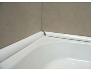
Score and snap profile - Clean with alcohol wipes and dry fit to tray to ensure they fit OK - Remove Strips and silicone tray with the large nozzle
