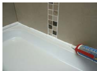
Fit profile one side at a time - push in at 45 degrees to get sealant up tiles and across tray base - Remove excess sealant with Fugi Tool or finger
