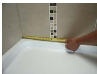
Measure tray internals and transfer measurements to profile - Mark and cut non profiled ends only
