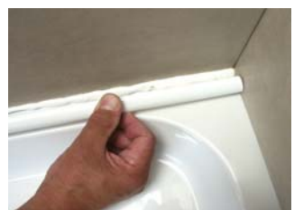
Fit profile one side at a time - push in at 45 degrees to get sealant up tiles and across tray base - Remove excess sealant with Fugi Tool or finger
