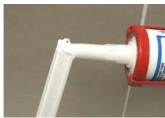
Fit profile one side at a time - push in at 45 degrees to get sealant up tiles and across tray base - Remove excess sealant with Fugi Tool or finger
