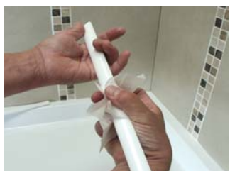
Score and snap profile - Clean with alcohol wipes and dry fit to tray to ensure they fit OK - Remove Strips and silicone tray with the large nozzle
