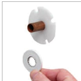
**3** Trim the projecting pipe to a length of 15-22mm, measured from the face of the gripper ring, using a rotary type cutter. If a hacksaw is used, the pipe end must be carefully de-burred and chamfered.
