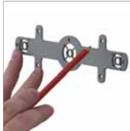
The template may also be temporarily secured to the wall to ensure correct orientation of the pipe work during making good if required.
