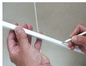
Measure length of bath and transfer measurement to 2m profile - Mark and cut to length by scoring and snapping profile - lay on bath "dry"
