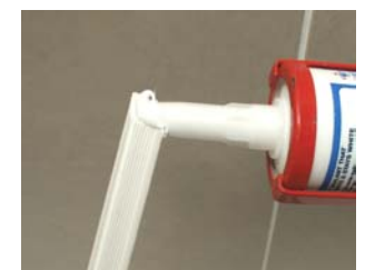
Clean Profile - Fit the long length 1st - Add generous silicone with large nozzle - Fit profile and remove excess with Fugi 2 or finger - Now fit end pieces
