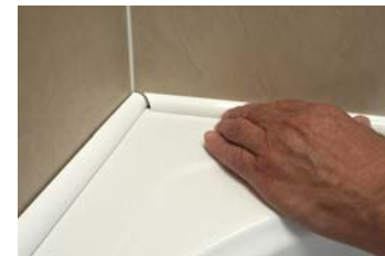
Take the appropriate 1m profile and fit it to the long profile behind taps - Mark to size - Cut and fit "dry" - Repeat with remaining profile
