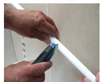
Measure length of bath and transfer measurement to 2m profile - Mark and cut to length by scoring and snapping profile - lay on bath "dry"
