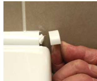
Change to fine nozzle - Seal in top and bottom of profile with silicon - Fit End Caps - Use Fugi 2 to remove excess silicone - Leave to Set ( 4 Hours )
