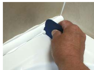
Clean Profile - Fit the long length 1st - Add generous silicone with large nozzle - Fit profile and remove excess with Fugi 2 or finger - Now fit end pieces
