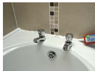
Clean Profile - Fit the long length 1st - Add generous silicone with large nozzle - Fit profile and remove excess with Fugi 2 or finger - Now fit end pieces
